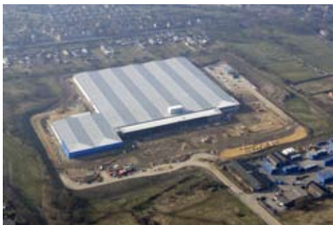
The new Thorns lighting factory in Spennymoor
