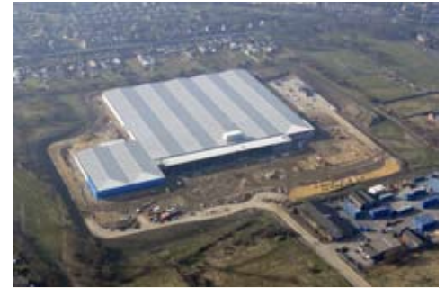
The new Thorns lighting factory in Spennymoor.
